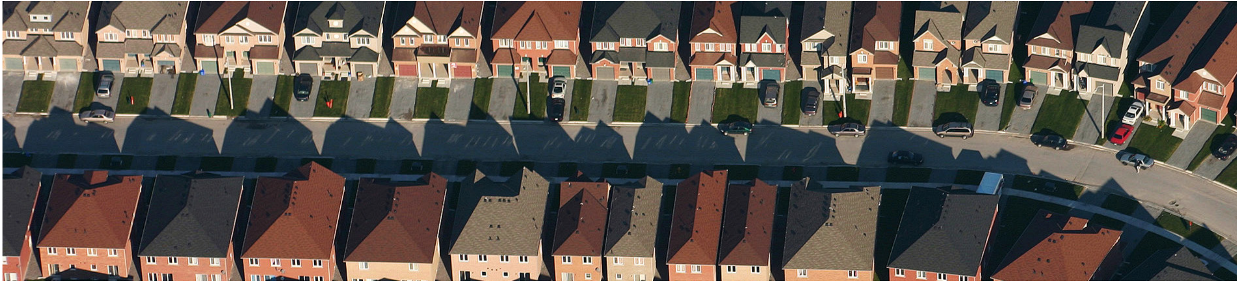
Picture: Housing developments in Markham, Ontario. (IDuke/Sting, 2005). CC BY-SA 2.5 [34]
