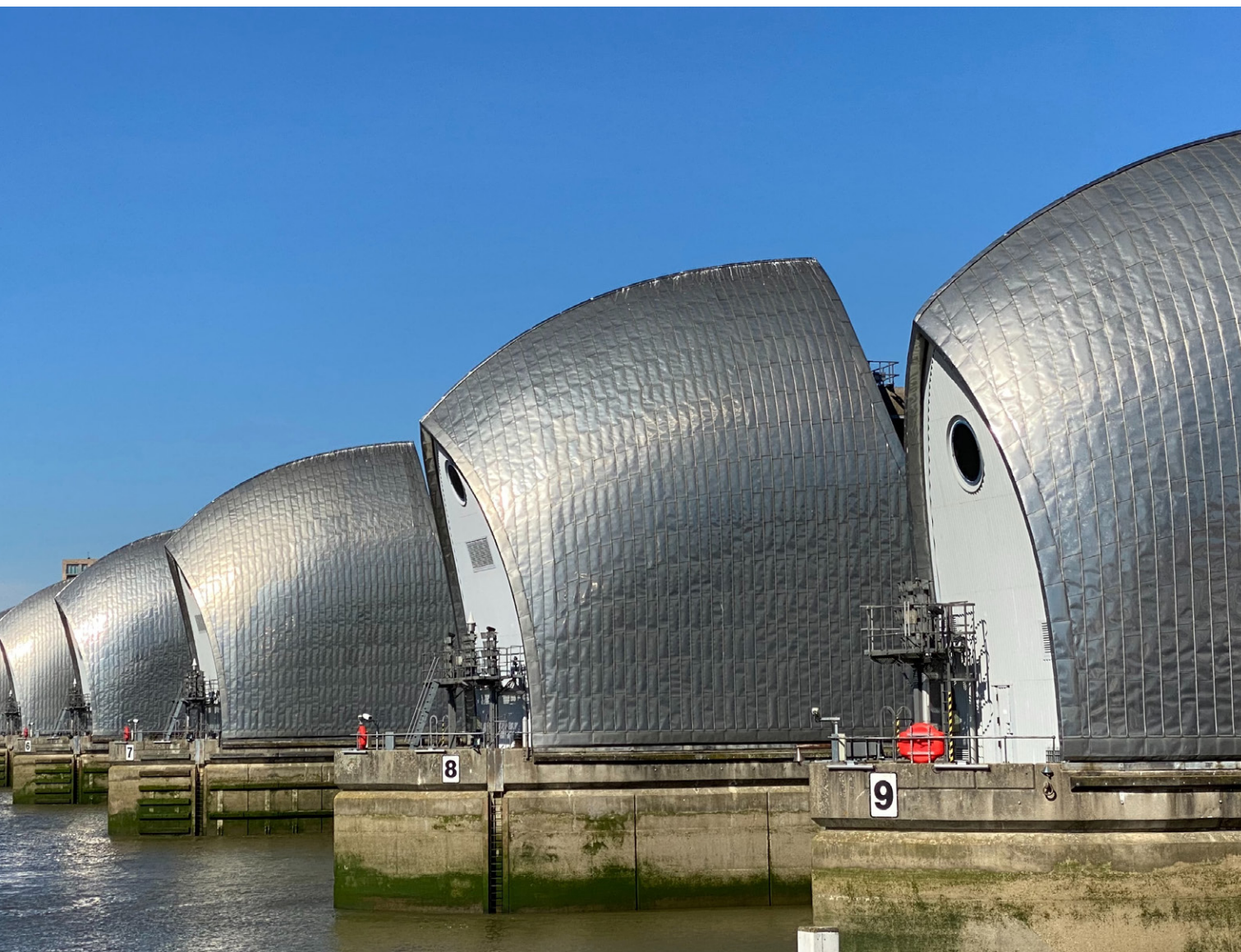
Pictured: The Thames Barrier in London, a retractable barrier system built in 1982 to protect the city from natural disasters such as flooding and storms. (Cameron, 2020) [77]
